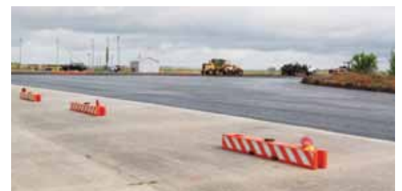
Dothan Regional Airport Authority and Commercial Jet Services, LLC recently celebrated the completion of a ramp improvement project at the airport.
